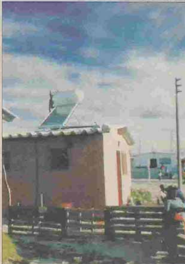
Elsie Tabalaza's house in Kuyasa is warmer than her neighbours' homes and she saves up to 40% on her electricity bill
